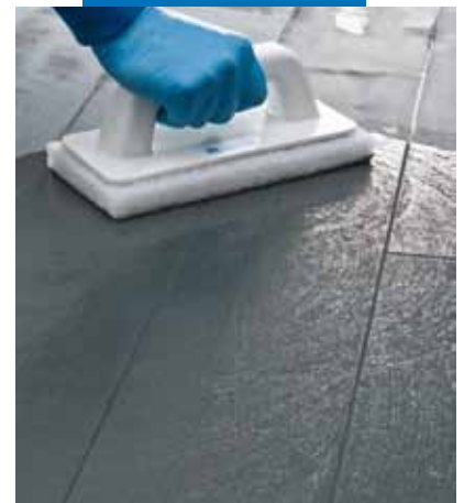
Cleaning the joints with a Scotch-Brite pad (when the product is semi hardened)
