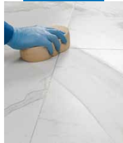
Cleaning and finishing the joints with a hard cellulose sponge
